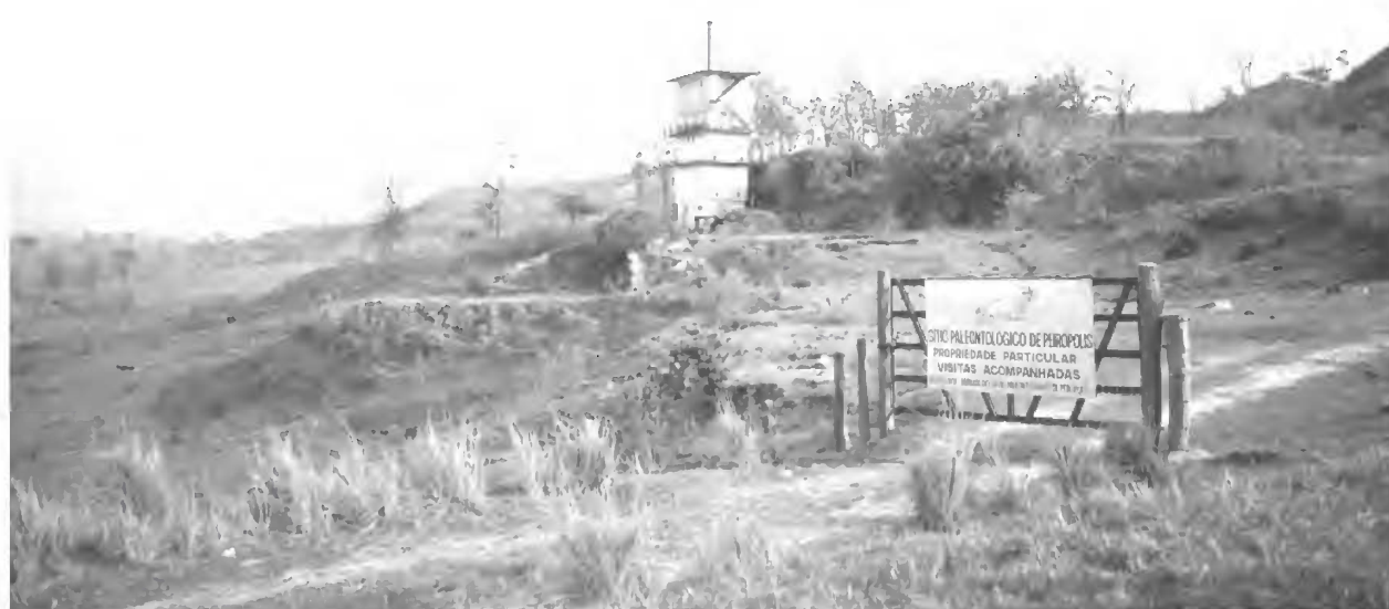
Fig.1- The Caieira site, near Uberaba, Minas Gerais State.
